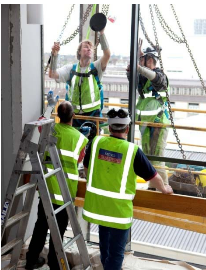
Figure 17: Glaziers repairing windows broken by the earthquake.
